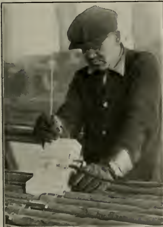
WELDER AT WORK WITH CASE COVERING THE ARC.
